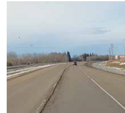
Longitudinal Joint Repair Before
