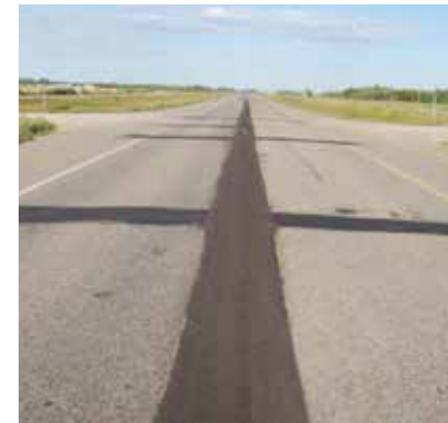
Longitudinal Joint Repair After
